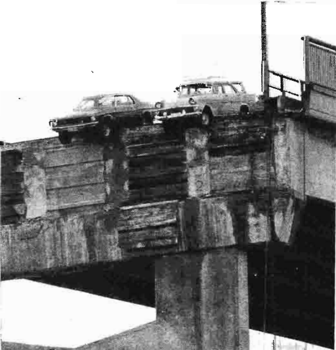
Two cars perched over the edge of the Tasman Bridge after an 80-metre span crashed into the River Derwent.
