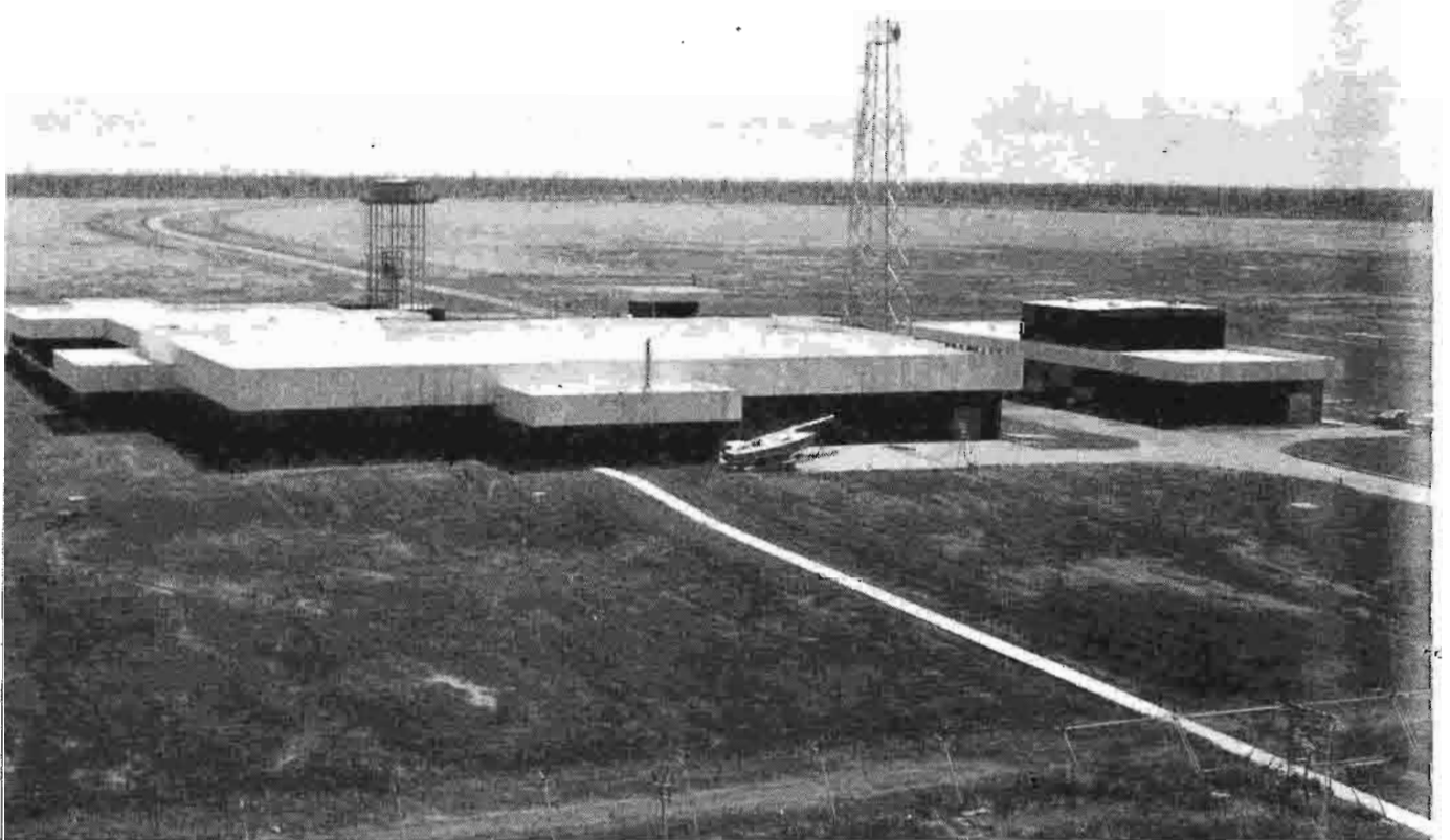
The new Naval Communication Station at Shoal Bay — though incomplete — went into makeshift operation when the cyclone put COONAWARRA temporarily "off the air".
