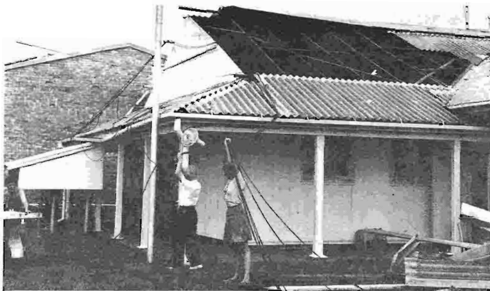
WRANS lend a hand with repairs at COONAWARRA.
