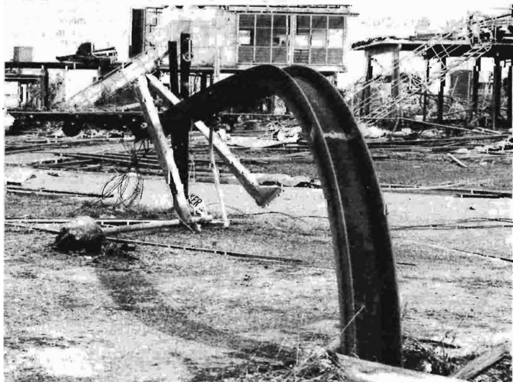
The bend in this steel telegraph pole, the uprooted road sign and what is left of these houses, gives some idea of the force of the cyclone.
