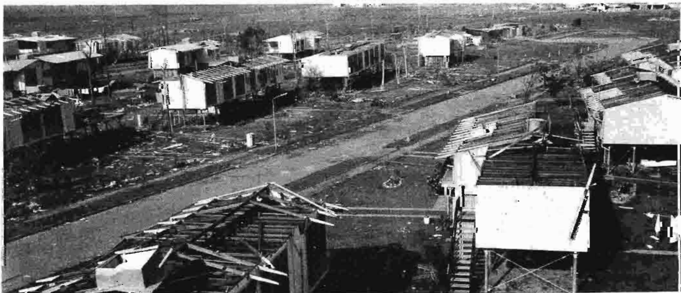
Some of the damaged Married Quarters at COONAWARRA.
