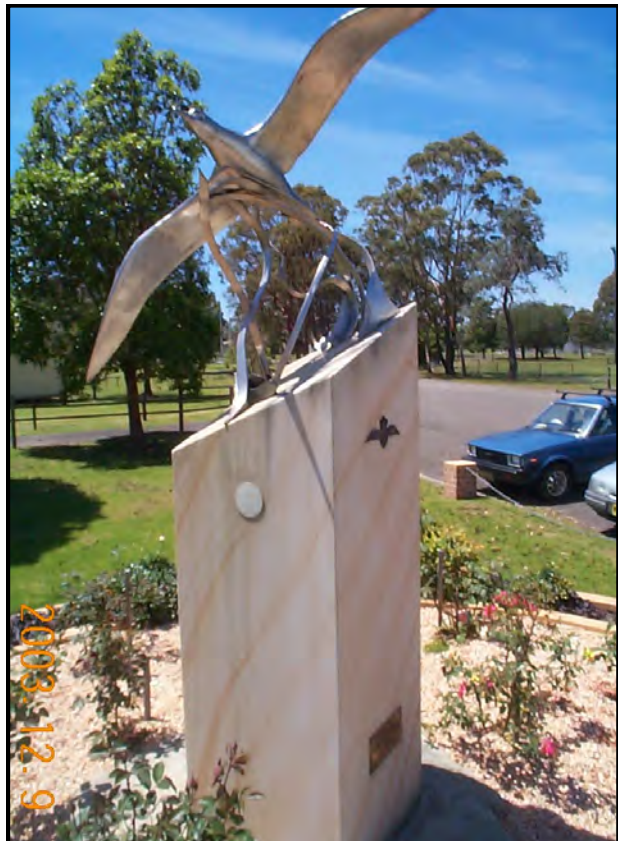
The sandstone plinth that the "Albatross" was mounted on suffered severe cracking as the result of the heat from the bush fires last year and the method used to affix it to the same. It was cracked on all four side and the top corner completely separated
