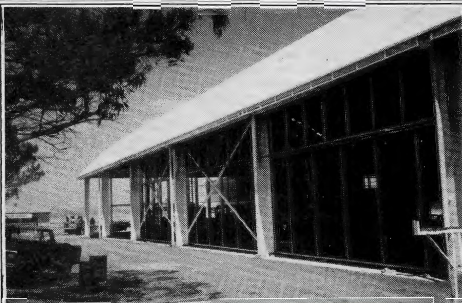
Museum walls under construction - January 1994
