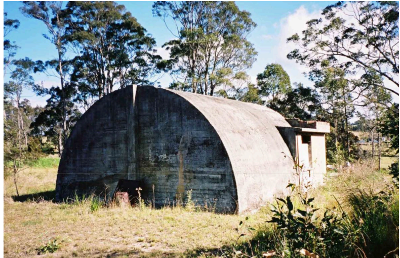
Above: One of the RAAF Torpedo Storage Bunkers at Nowra, just off BTU road. (Image: acomos.com ).
