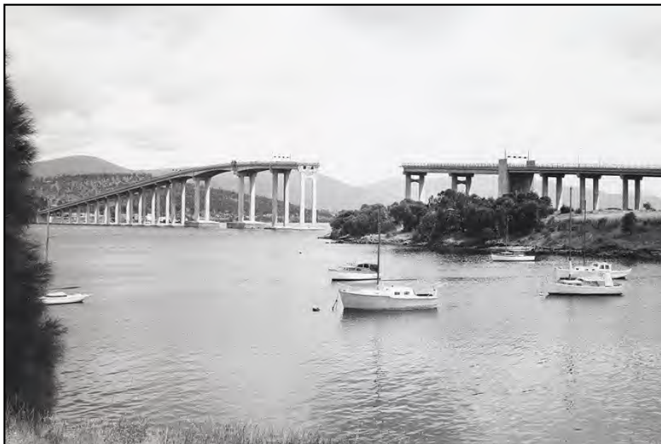
Tasman Bridge after the Lake Illawarra hit the pylon with part of the bridge collapsed on the ship, sinking it.
