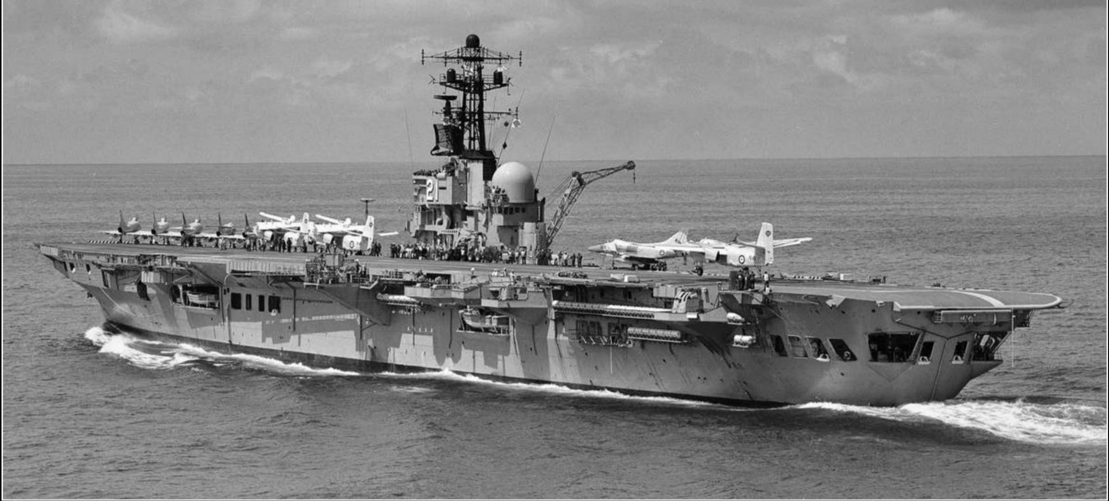
Above. Looking spick and span, HMAS Melbourne steams on a calm ocean whilst operating her new aircraft. A Tracker is about to capture an arrestor wire, whilst other Trackers and Skyhawks are secured in the parking areas forward and aft of the island. Once again, this photo illustrates how little room there was to operate modern aircraft aboard a light fleet carrier. (Photo: Fred Tyler). ➔
